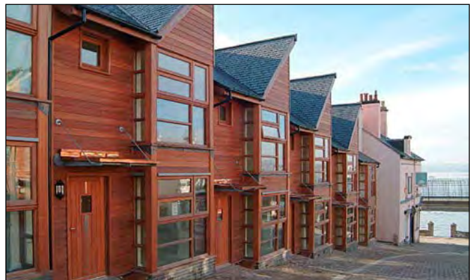
Fig 5.11: This development responds well to the sloping site and views out by stepping buildings down the slope and orienting the street to open up to the waterside
